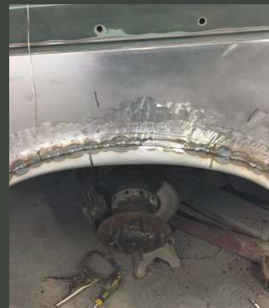
The inner rear arches needed replacing along with the outers, with RS Bodywork being entrusted to carry out the repairs
